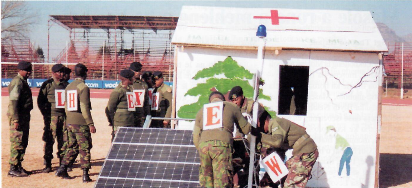
Litho tsa lebotho la Engineering li hokahanya lithapo tsa phepelo ea motlakase oa matla a letsatsi setsing sa kokelo.
